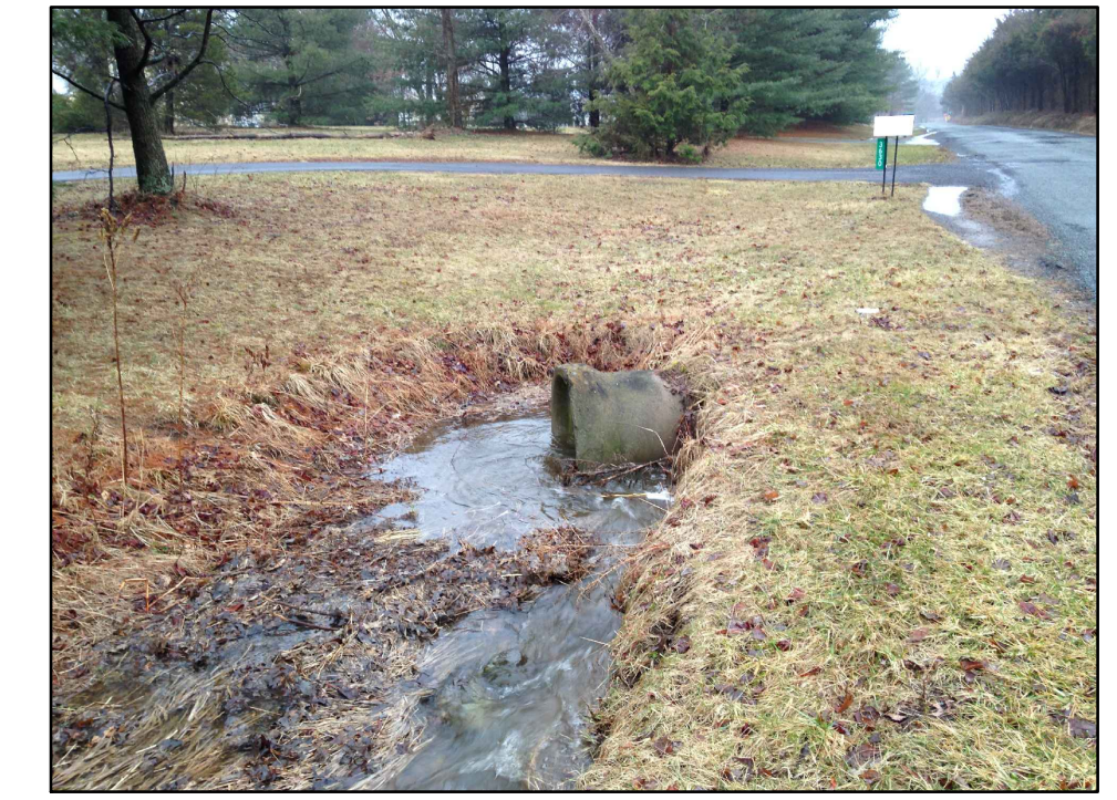
EX. CULVERT #4 PHOTO. 2 NOT TO SCALE, LOOKING SOUTH
